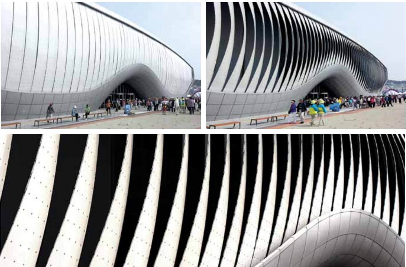
Fig.22-24: Kinematic facade of the Thematic Pavilion EXPO 2012 in Yeosu, South-Korea. Architects: soma-architecture, Vienna; Engineer for Kinetic Facade: Knippers Helbig, Stuttgart, New York.
