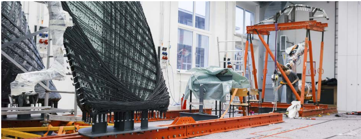
Figure 8: Formwork system of the cantilever (left to right): portal frame and permanent part of the structure, temporary tip frame with push-pull props and steel extension
